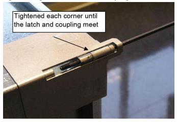
Figure 27: Properly Installed Filter Inside of the Frame
