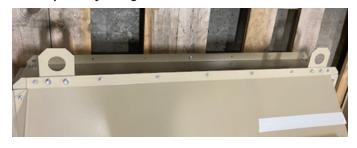
Figure 87: Bottom flange of hood screwed to unit while held in place by lifting bracket
